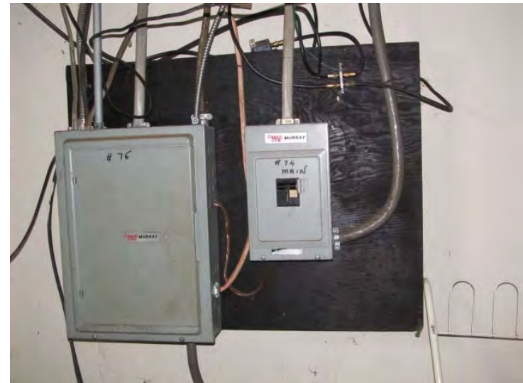
Main electrical shut-off (breaker) for some units is located in the basement of the adjacent unit at some buildings
