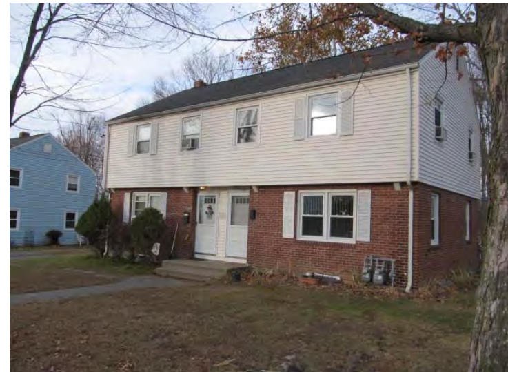
Some buildings feature brick veneer on the exterior walls at the first floor level
