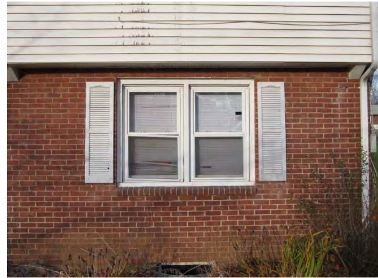
Typical aluminum-framed windows with double glazing
