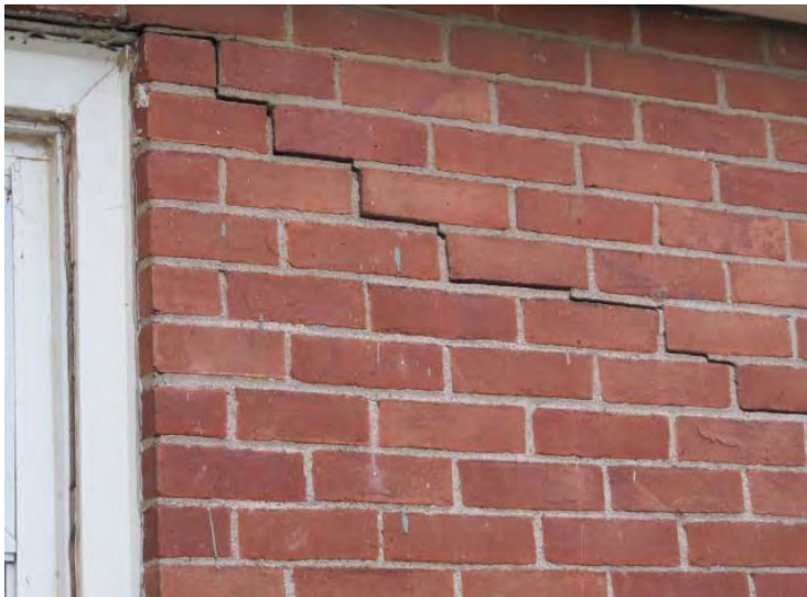
Isolated step crack noted in brick veneer
