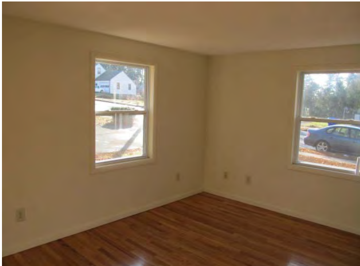
Original wood strip flooring in unit living areas are in good overall condition
