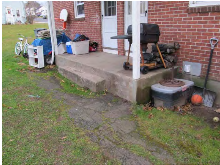
Asphalt walkways leading to unit entries are narrow and exhibit high levels of wear/deterioration at various locations
