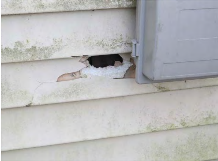
Dirt and organic growth typical on vinyl siding surfaces – Age related wear and impact damage also noted at some locations
