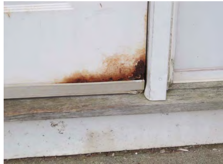
Rust damage noted on several of the common entry doors
