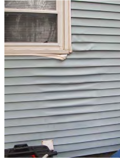
Heat damaged vinyl siding – Some siding Colors are no longer available which prohibits cohesive repairs
